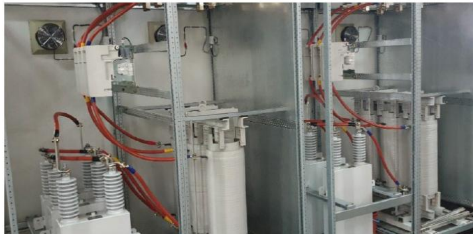
11kv IP42 Indoor Bank with Detuned Reactors
